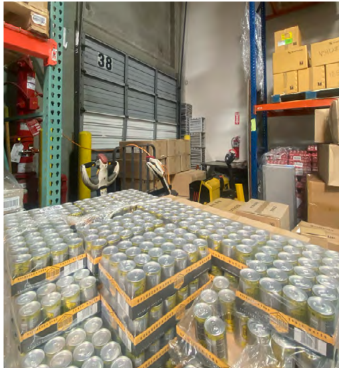
Pallets and boxes blocking access to fire extinguisher and exit
